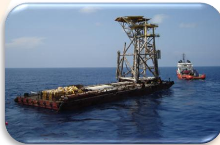
Unmanned platform abandonment
