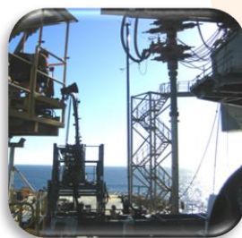
CT-ESP installation concurrent to drilling
